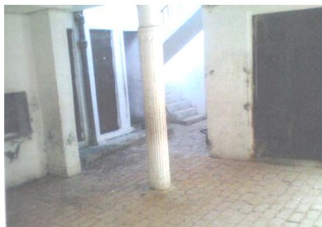
Figure 3: Interior view of residential building that is being used as School 2
